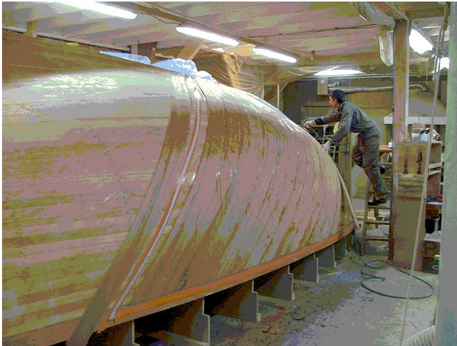
Pictured is the Finistere under construction in July 2008.
